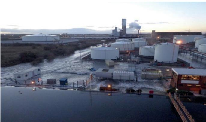
ABOVE: Inter Terminals, Riverside Terminal. Water overtopping the flood defences – as seen from a ship at the terminal. BELOW: SABIC Brinefields and Cavities storage area showing the flood defence breach. © Environment Agency
